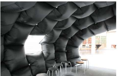
Inflatable folly for in- and outdoor video presentations. The folly creates a separated dark space in a larger envirement. The construction consists of connected individual airbags. The different shaped bags and the pressurized air inside give the tent its shape and firmness. The construction leans against the wall which can be used as a projection screen. Commissioned by:CBK GroningenYear of completion:2008Exposition locationsGroningenMilan2009St. Etienne2009
