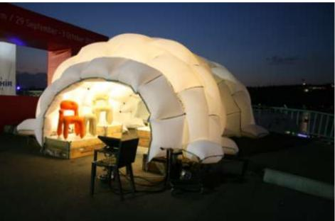
Inflatable tent for indoor and outdoor events. The tent consists of over one hundred connected individual airbags. The different shaped bags and the pressurized air inside give the tent its shape and firmness. Commissioned by: Year of completion: Exposition locations: own development
