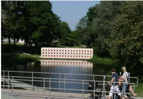
The Air Bridge has been developed as a test object to examine the possibilities of inflatable spans. The results are still to be incorporated into an inflatable building with multiple floors. The construction consists of only pressurized air and cloth.
